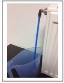
During the bleeding process, we recommend draining the escaping airwater mixture into a suitable container.
