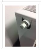
First disassemble the factory-fit ECO air vent.
